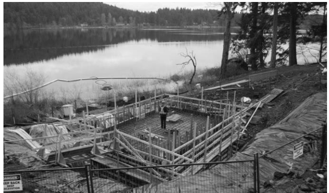
Preparing to pour concrete slab for the intake tower.
