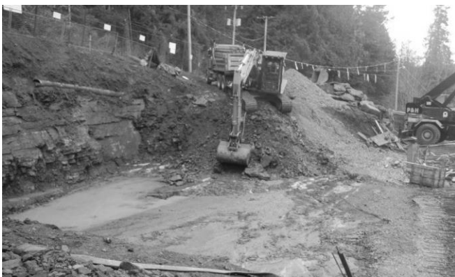
Evacuation in progress for process room slab.
